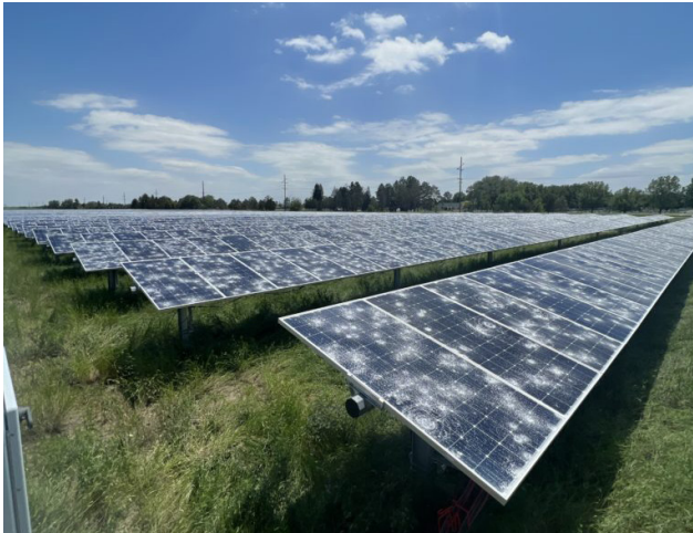
Hail severely damaged a solar farm on June 23, 2023. (Courtesy: Nebraska Public Power District)
