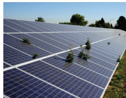
Figure 4 — Vegetation growth in a fixed-tilt system
